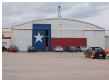
The hangar, pictured above, is a fitting place to construct a truly Texan entry for the Solar Decathlon competition.
