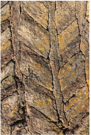
TURF WALL Shown here is the outer layer, stacked in herringbone pattern. Each of the three layers of the wall's section are cut using specialized tools and regionally specific technique.
