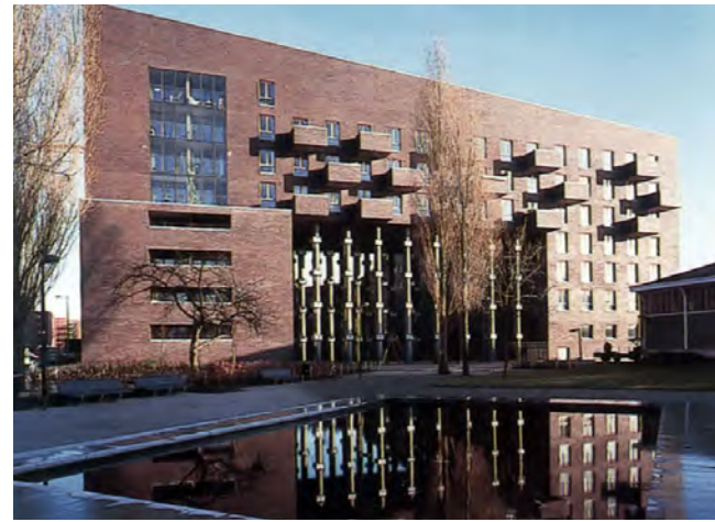
Transparent gate façade
