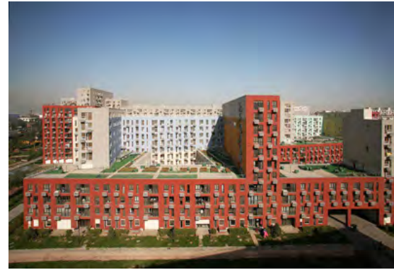
Exterior view looking north
