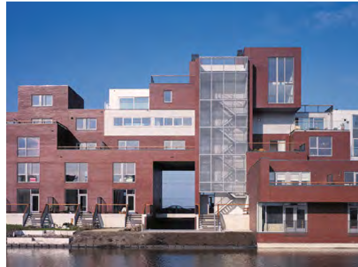
Exterior detail: portal from canal
