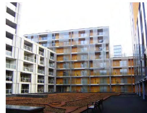
View from courtyard
