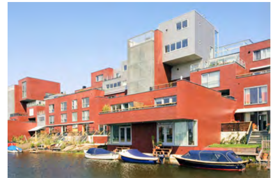
Exterior view from canal
