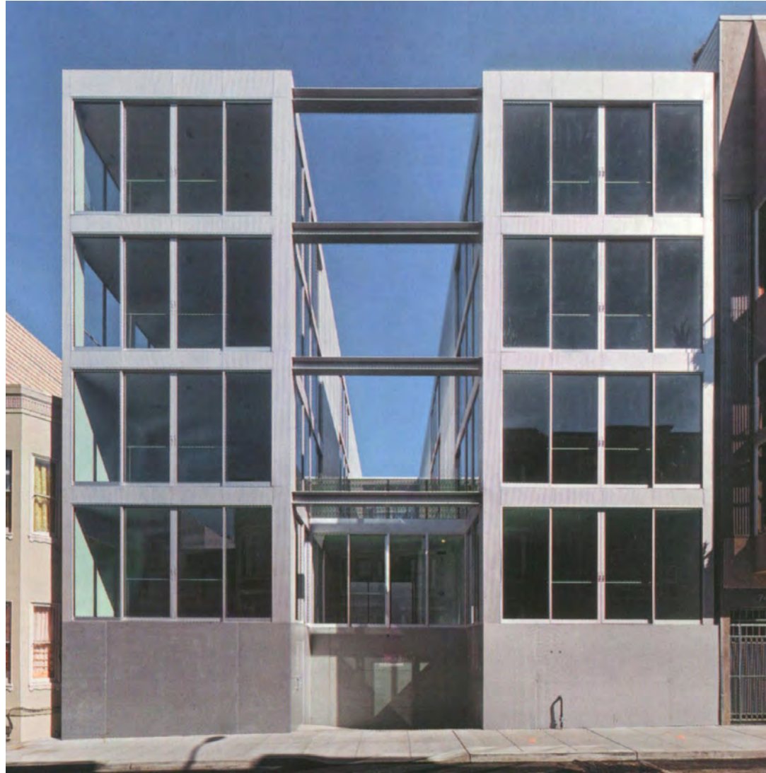
Natoma Street facade
