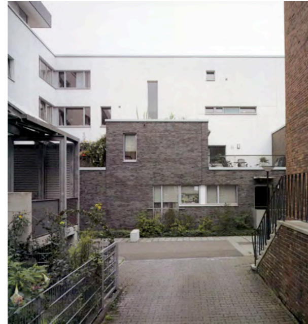
Facing eastern facade
