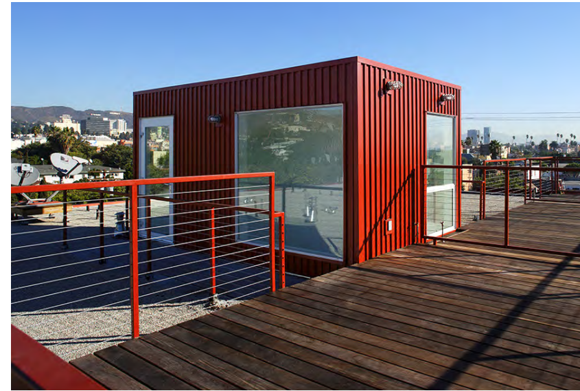
Rooftop access point
