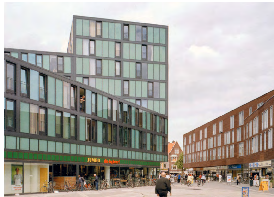
Exterior view of courtyard
