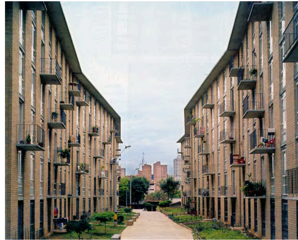
View between housing blocks
