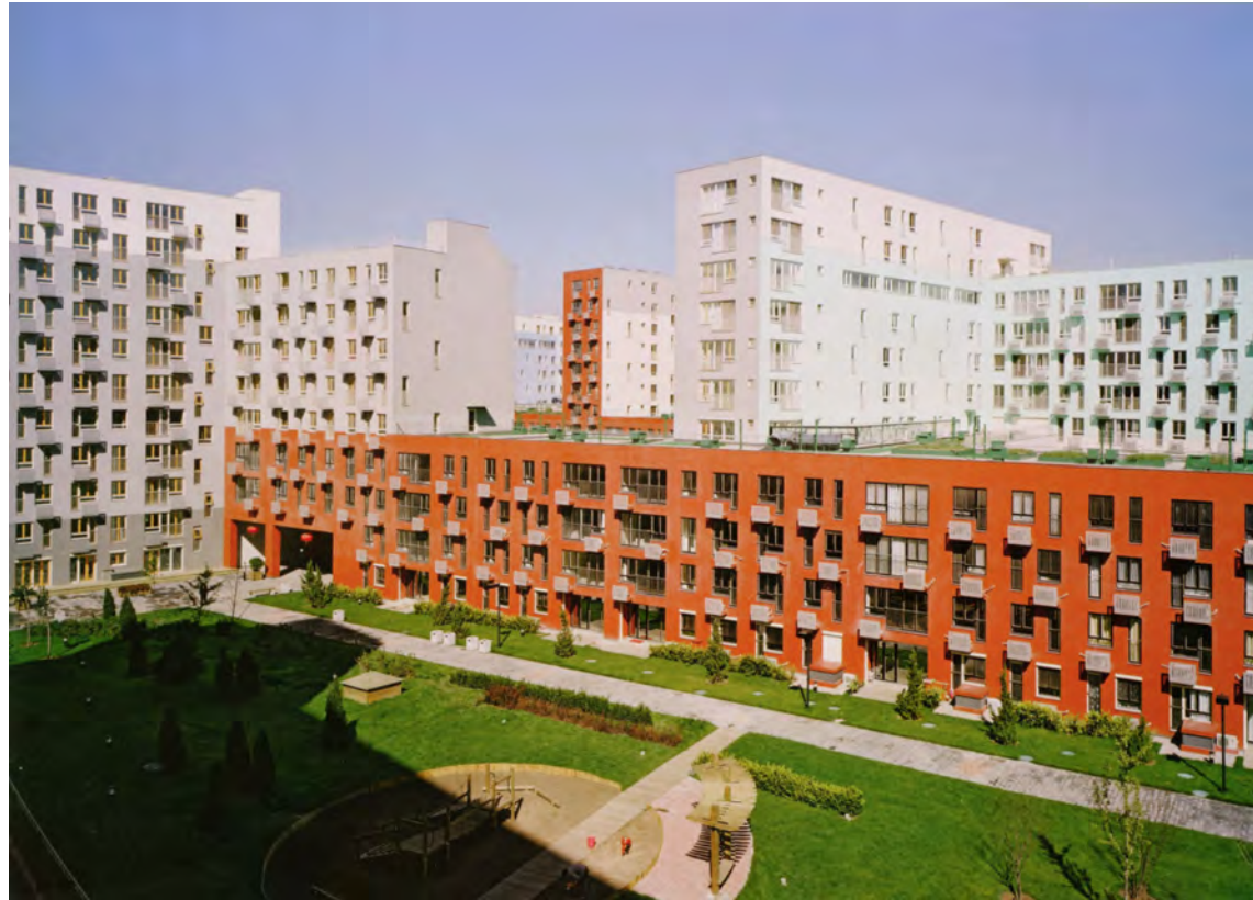
Exterior view of courtyard looking south
