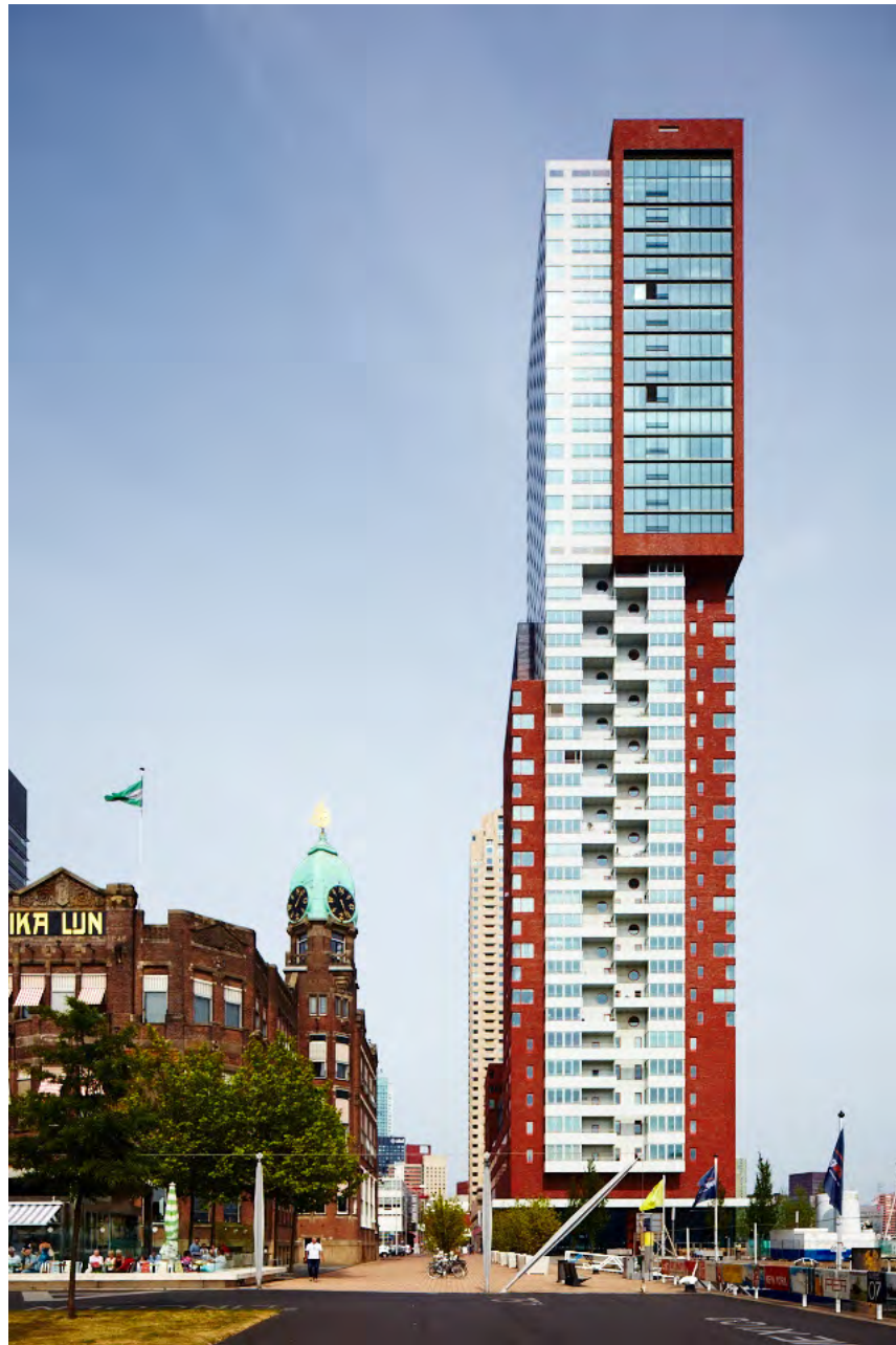
View of tower
