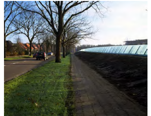
View looking north
