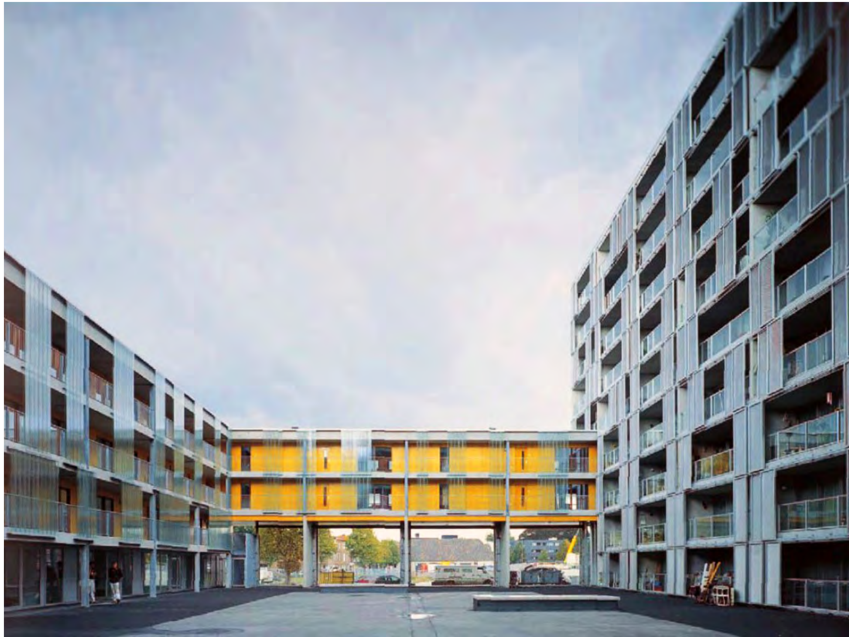
View from courtyard looking north
