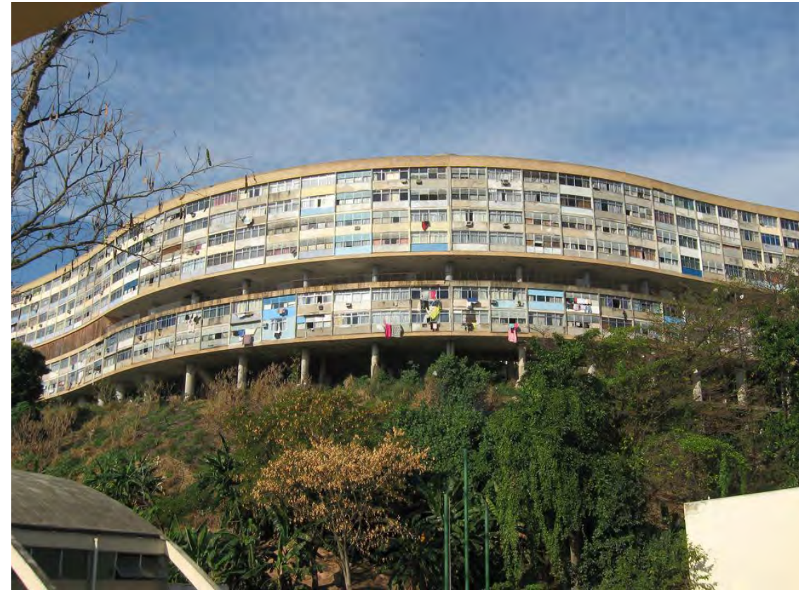
Exterior views: current condition
