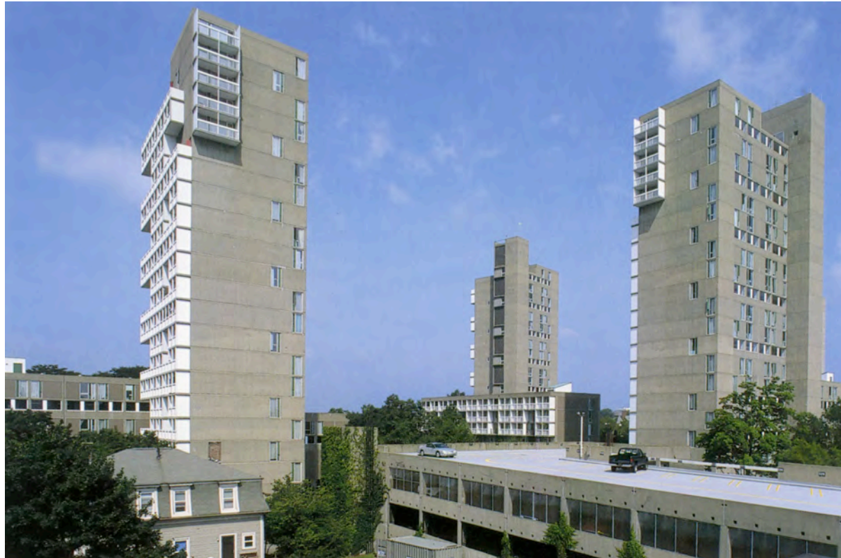
View of towers to the northwest
