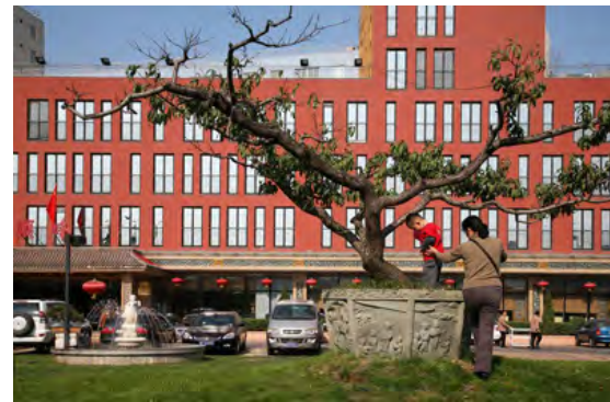
Exterior view of courtyard looking south
