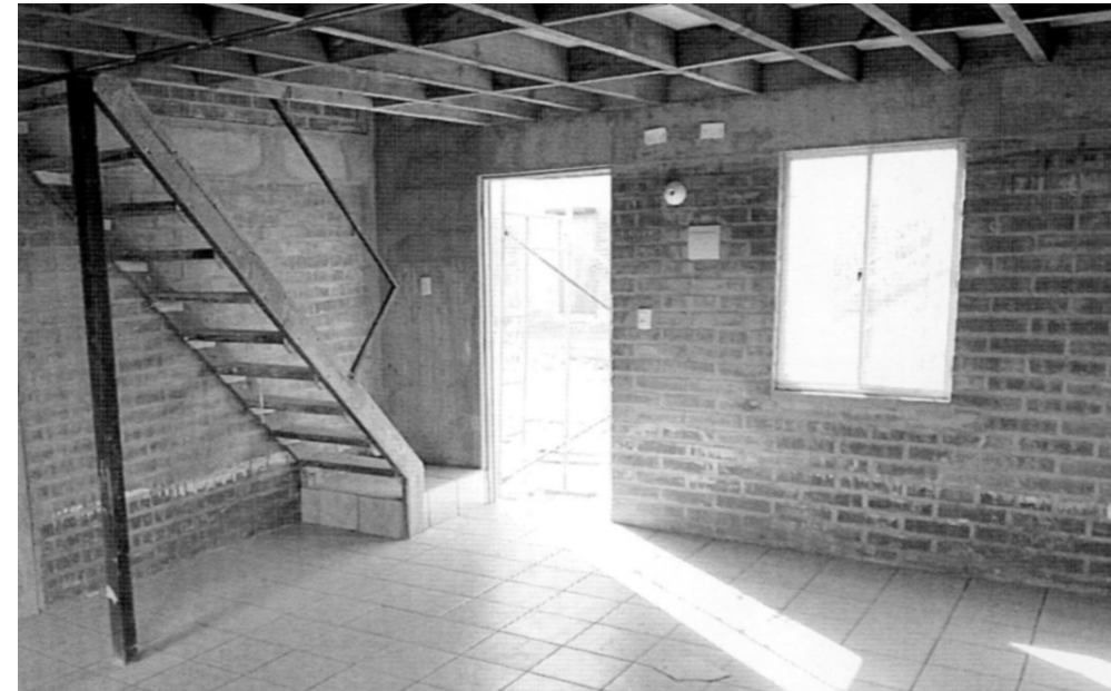
Interior view: shell
