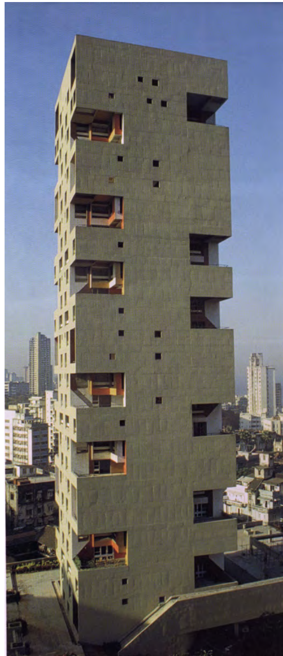
View of tower
