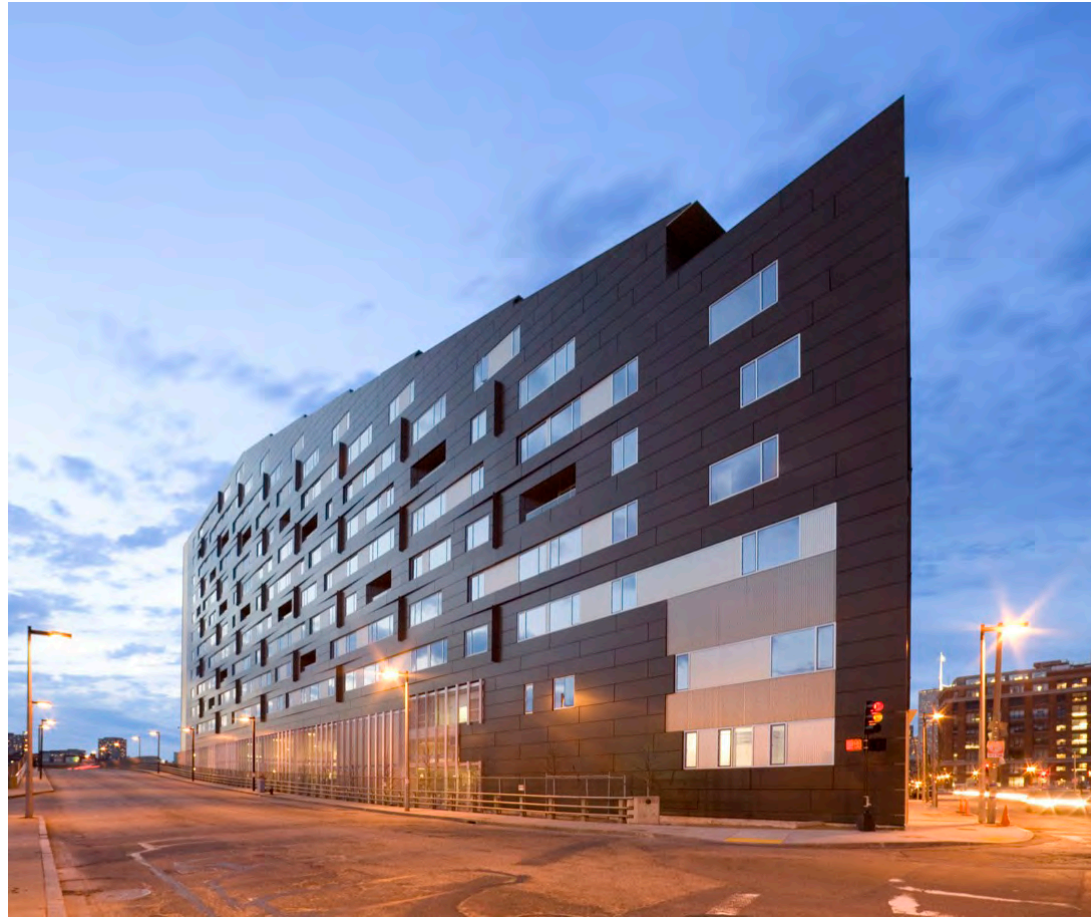
Expression of structural system and unit module in the façade articulation
