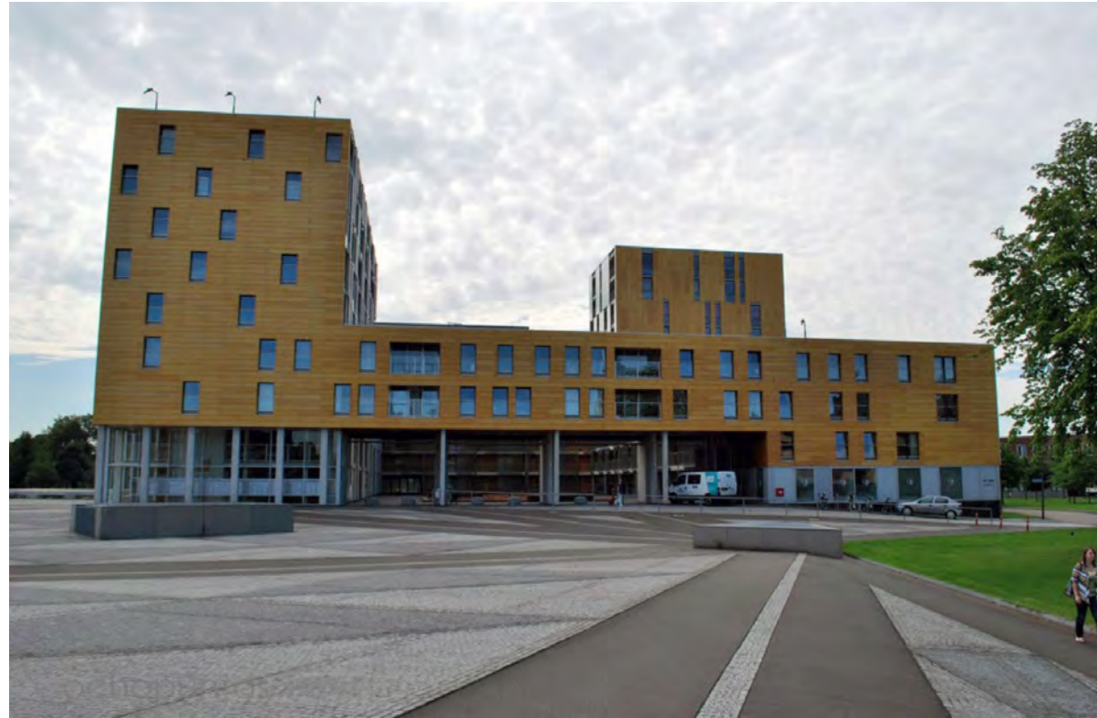
Transparent façade (north)
