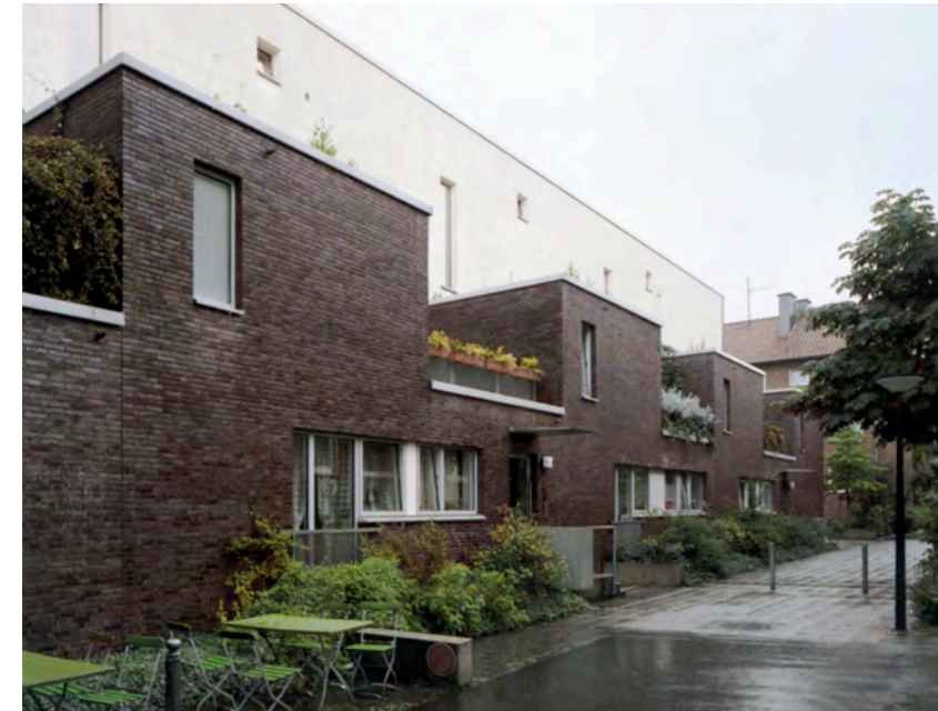
Facing south down access road
