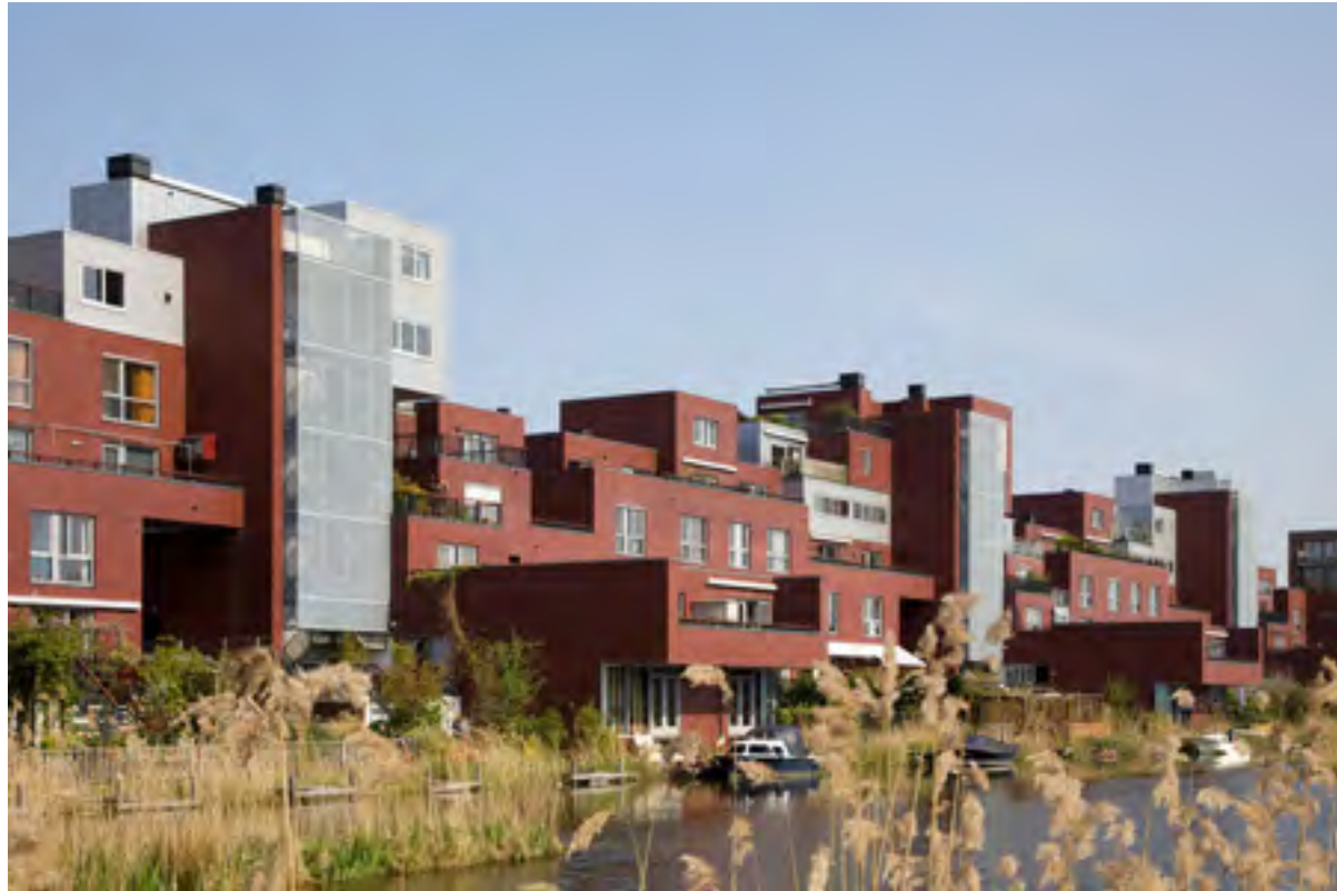
Exterior view from canal
