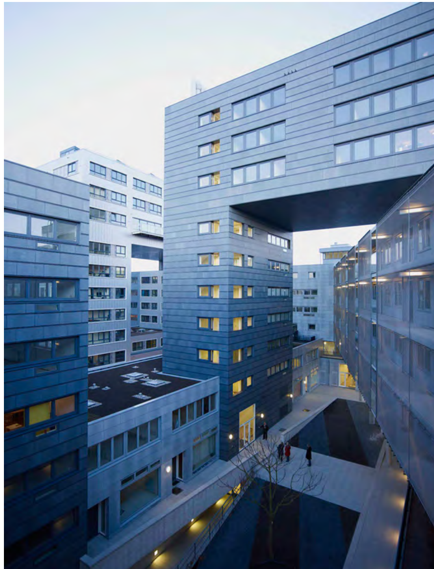
Exterior view of courtyard
