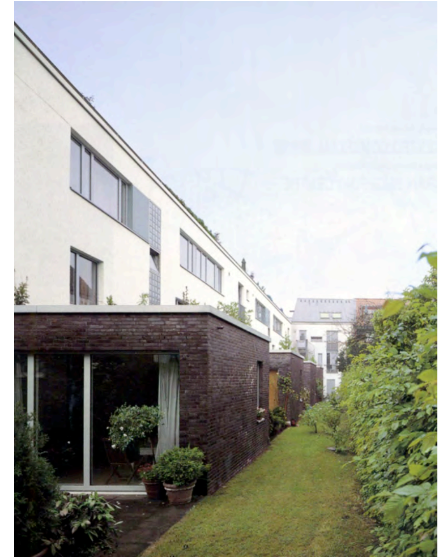
Western edge of building
