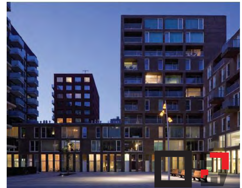
View from inside the courtyard
